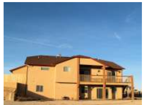
Back Side Upper Deck & Lower Patio. This Illustrates How Big Home Really Is.
